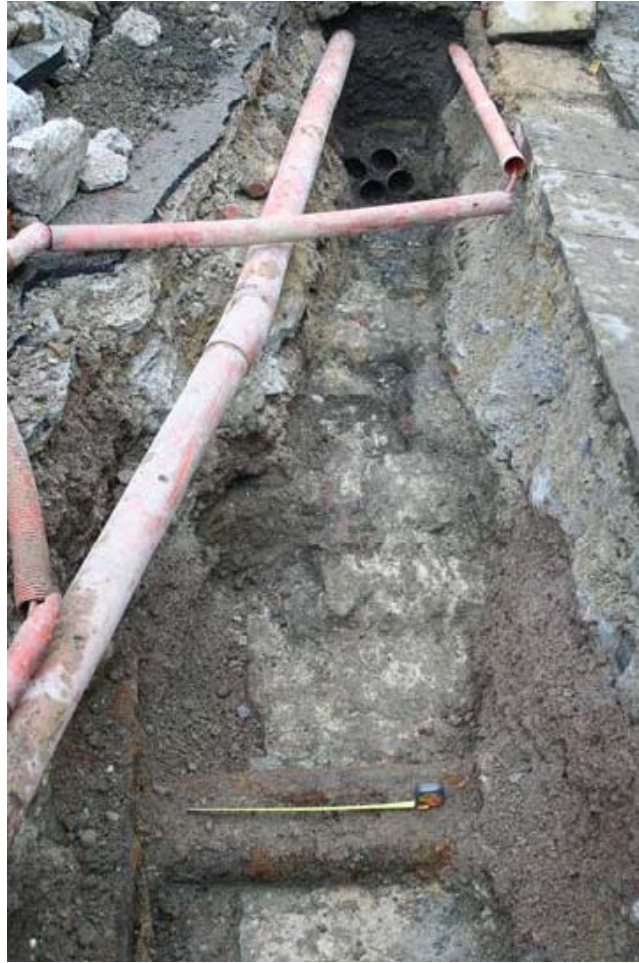
Figure 8: Base of the London Wall disturbed during TFL works at Aldgate. (Image: Historic England)
